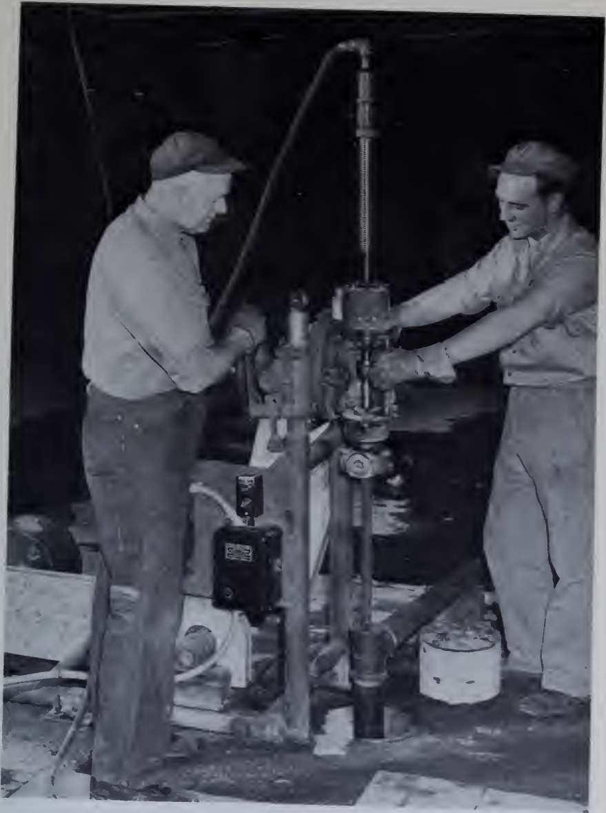
Figure 207.—Drilling a 10-inch core in concrete floor. PX-D-33518.
